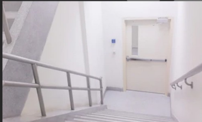
Self-closing stairwells, preventing access to alternate floors
